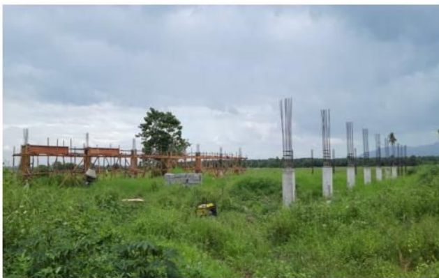
Title: Construction of Gymnasium Location: Lutayan Campus ABC (Php): 7,000,000.00
