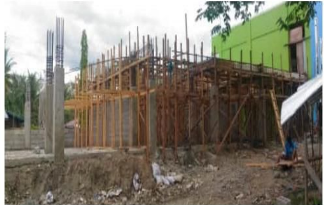
Title: Construction of Academic Building Location: Kalamansig Campus ABC (Php): 8,000,000.00
