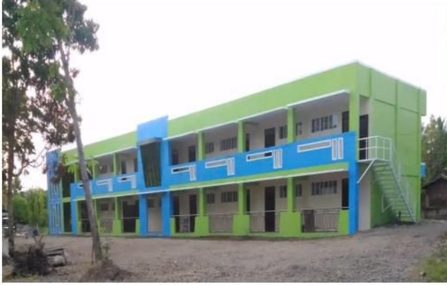
Title: Construction of Academic Building Location: Kalamansig Campus ABC (Php): 10,000,000.00
