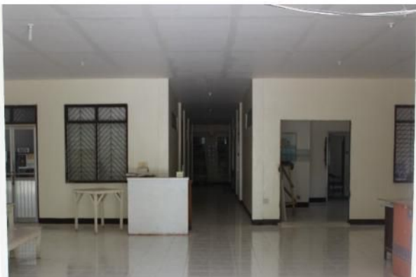
Title: Repair of Nursing Building Location: ACCESS ABC (Php): 2,500,000.00
