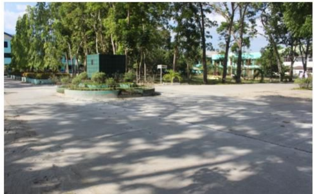
Title: Construction of Road Pavement Location: ACCESS ABC (Php): 800,000.00
