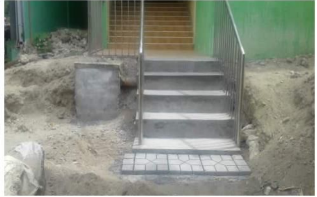
Title: Repair of Stairs for Birthing Clinic Location: ACCESS ABC (Php): 26, 812. 35
