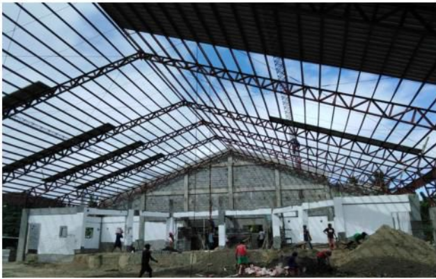
Title: Construction of Gymnasium Location: Kalamansig Campus ABC (Php): 7,000,000.00
