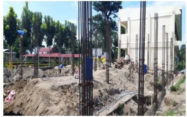
Title: Construction of Academic Building Location: Lutayan Campus ABC (Php): 7,000,000.00
