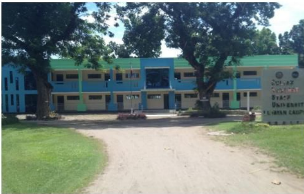
Title: Construction of Academic Building Location: Lutayan Campus ABC (Php): 10,000,000.00
