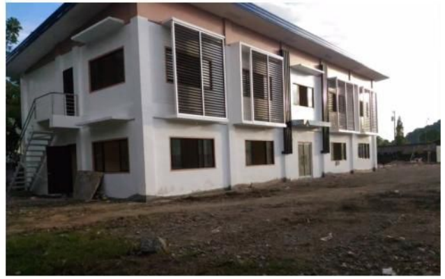
Title: Construction of Dormitory Location: Kalamansig ABC (Php): 5,000,000.00
