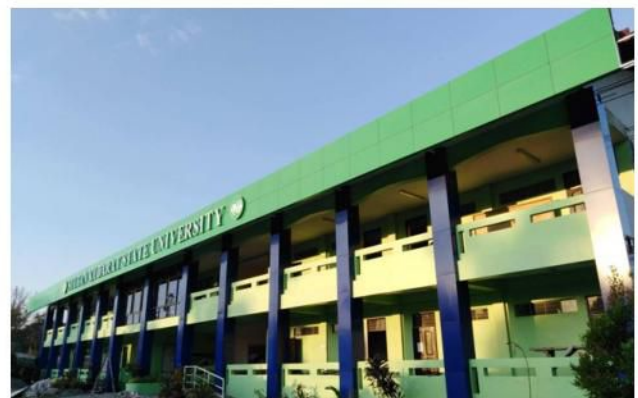
Title: Repair/ Rehabilitation of Two-Storey Academic Building (Front Building) Location: Tacurong Campus ABC (Php): 1,484,262.62
